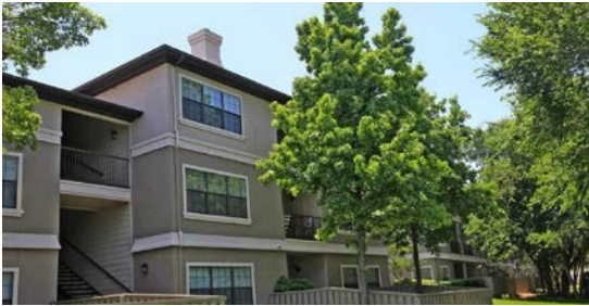
Verandas at Timberglenn
